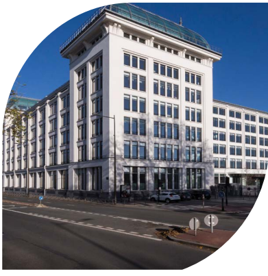
IN & OUT (SCI BOULOGNE LE GALLO) Boulogne-Billancourt (92)
